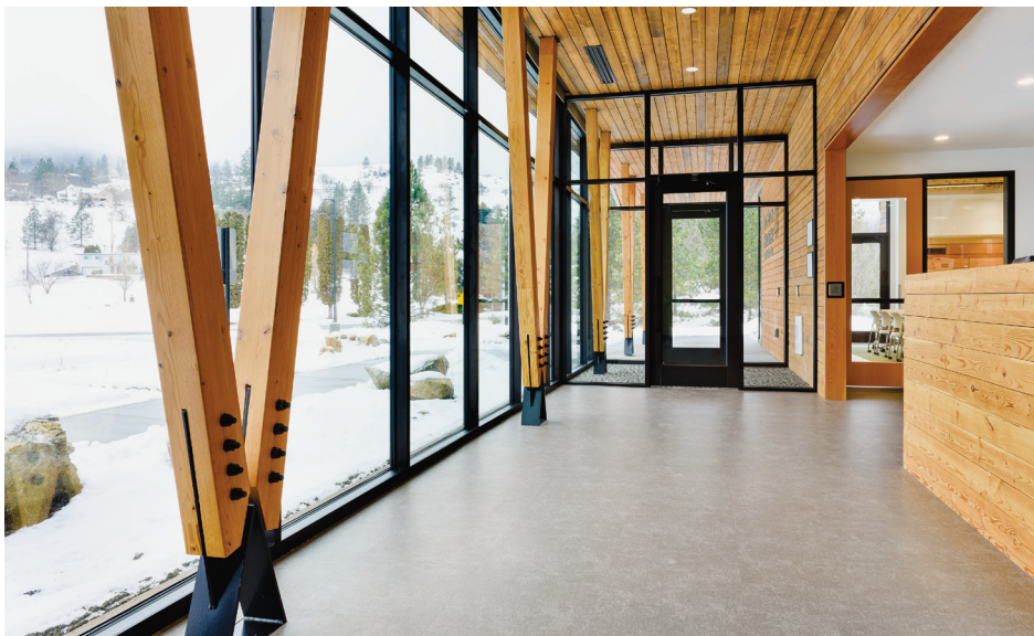
Nez Perce-Clearwater National Forests Supervisor's Office – Kamiah, ID USDA U.S. Forest Service, Mosaic Architecture, Morrison-Maierle / Two-story hybrid of mass timber and light-frame wood
