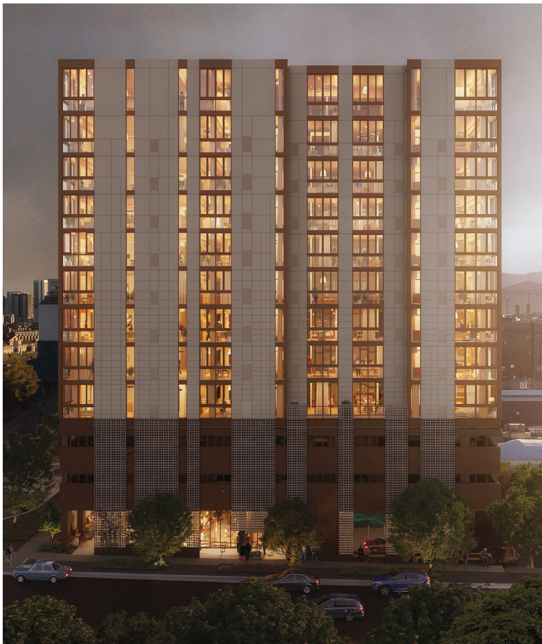
Return to Form – Denver, CO Katz Development, tres birds, KL&A Engineers & Builders
